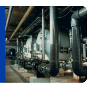
Durapipe PVC-U has been used for the conveyance of water, effluents, acids and chemical concentrates within different industrial applications for many years.
