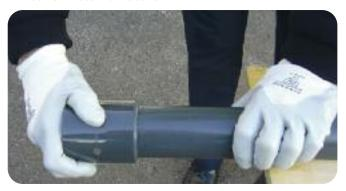
7. Wipe off excess cement from the outside of the joint.
