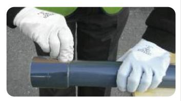
8. Using the mark previously made, check that the pipe has been fully inserted.
