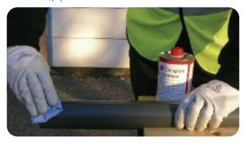
Using a clean brush, apply cement to the pipe and fitting.The joint surfaces should be completely covered by cement.
