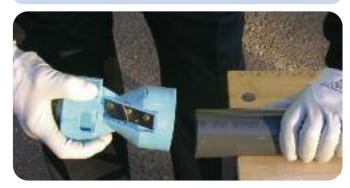
Remove any dirt, grease or moisture. A thorough wipe with a clean, dry rag is usually sufficient. Check dry fit. Pipe should insert easily into socket, approximately  $^{1}$ /4 to  $^{3}$ /4 of the total socket depth.
